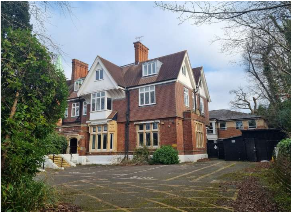
EXISTING BUILDING ENTRANCE VIEW
